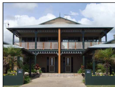
Examples of good balcony/verandah design
