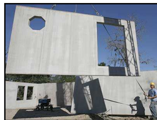
Prefabricated Concrete Panel
