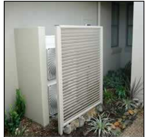
An example of an air-conditioning screen located at ground level (Sourced from: spec-net.com.au )
