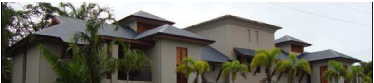
This roof design provides a good example of the use of large eaves and a staggered roof profile to break up the bulk of the roof. The roof is also constructed using Colorbond sheeting.
