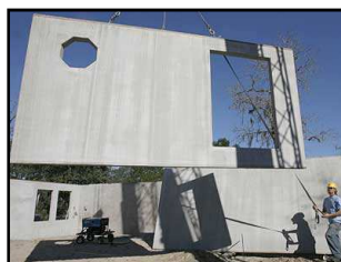
Prefabricated Concrete Panel
