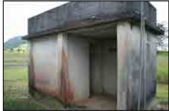
Laundry/bathroom topped with water tank
