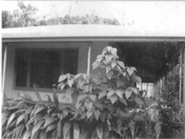
Ninney Rise - view of house from south, including veranda
