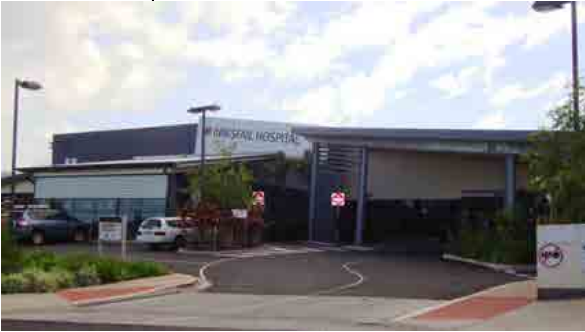
New section of hospital built in the 1990s
