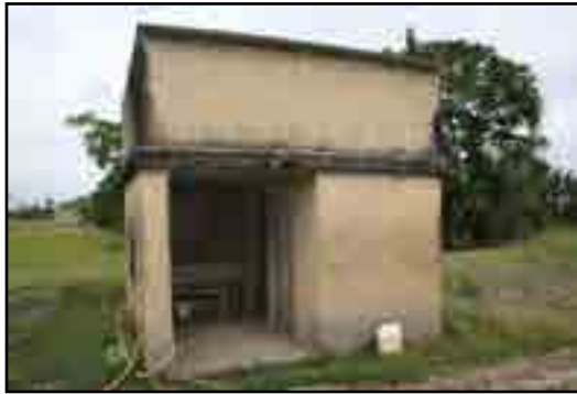
Laundry/bathroom with water tank on top
