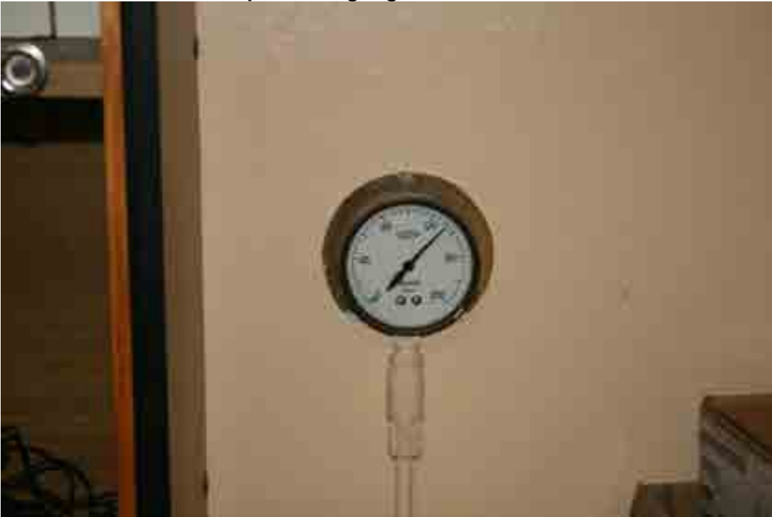
Downstairs town water pressure gauge
