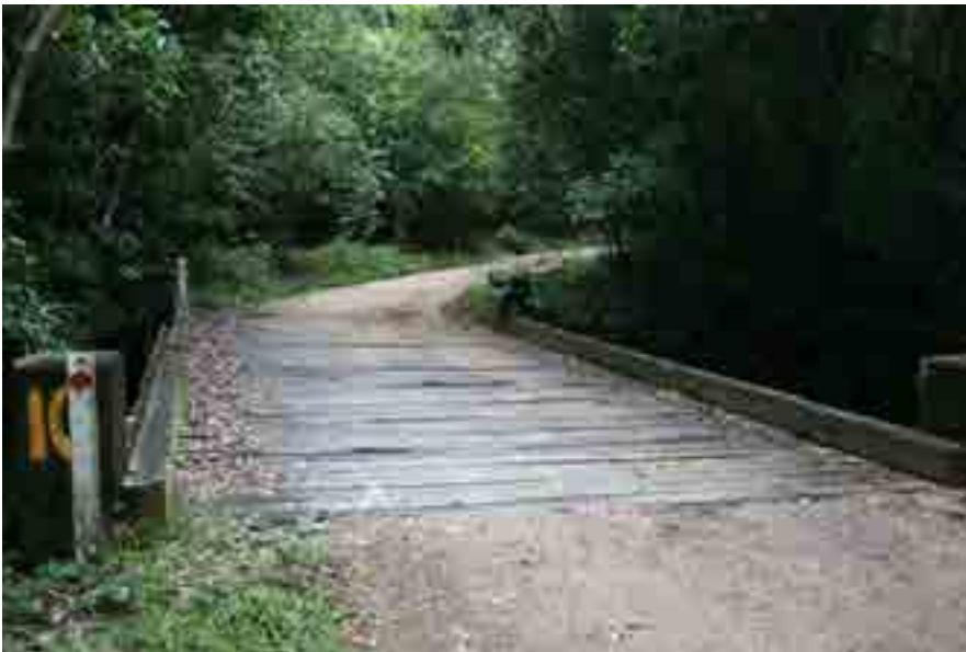
Kirrama Range Road: Bridge 10
