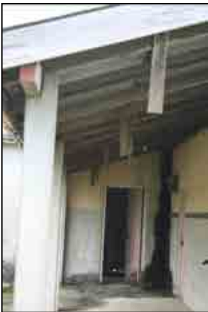
Verandah still has clothes line, hooks and paint work
