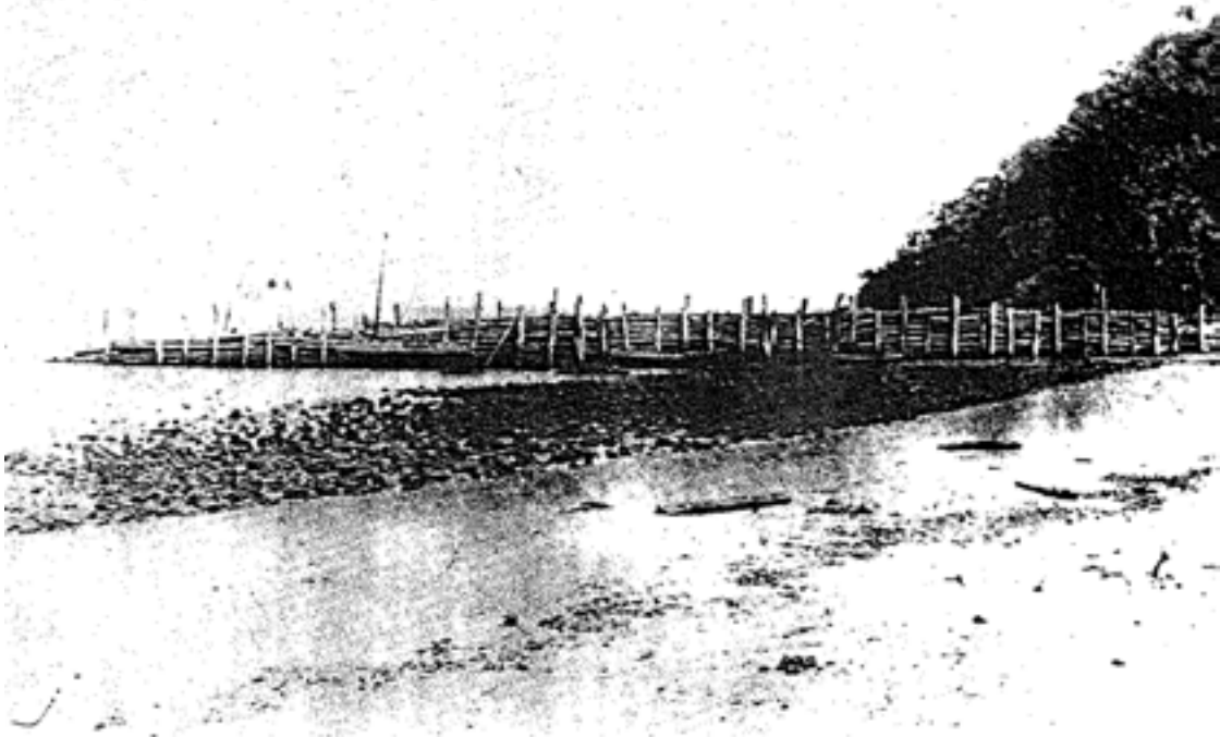
Breakwater, Cutten Coconuts, 1895, Taylor pg.10
