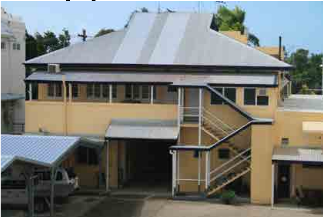
Rear of building - original section
