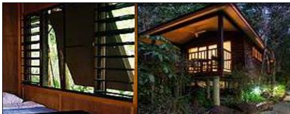
Example of awnings comprised of timber battens to encourage shade and protect openings (Images sourced from: http://www.thalabeach.com.au/port-douglas-accommodation/ http://www.capetribbeach.com.au/cape_tribulation_accommodation.htm )
