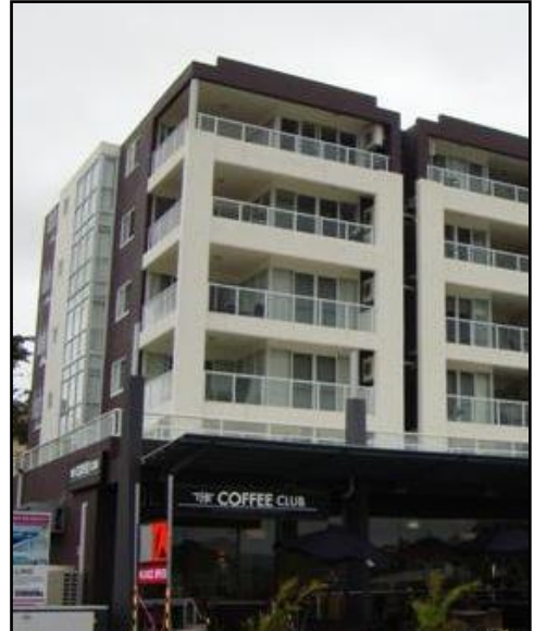
The River Grande incorporates commercial uses on the ground floor.
