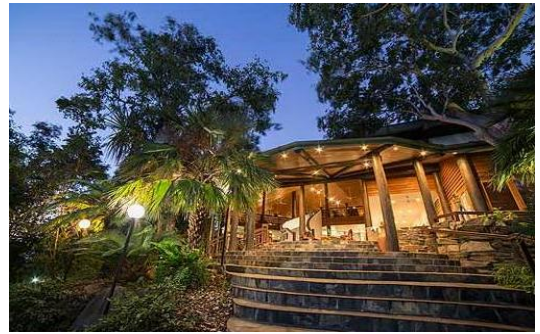
Examples of external light being minimised to reduce off-site illumination and light pollution (Images sourced from: http://www.thalabeach.com.au/ )
