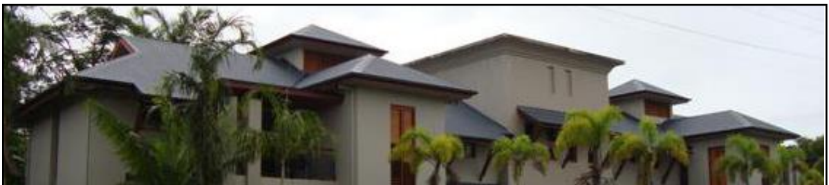
This roof design provides a good example of the use of large eaves and a staggered roof profile to break up the bulk of the roof. The roof is also constructed using Colorbond sheeting.
