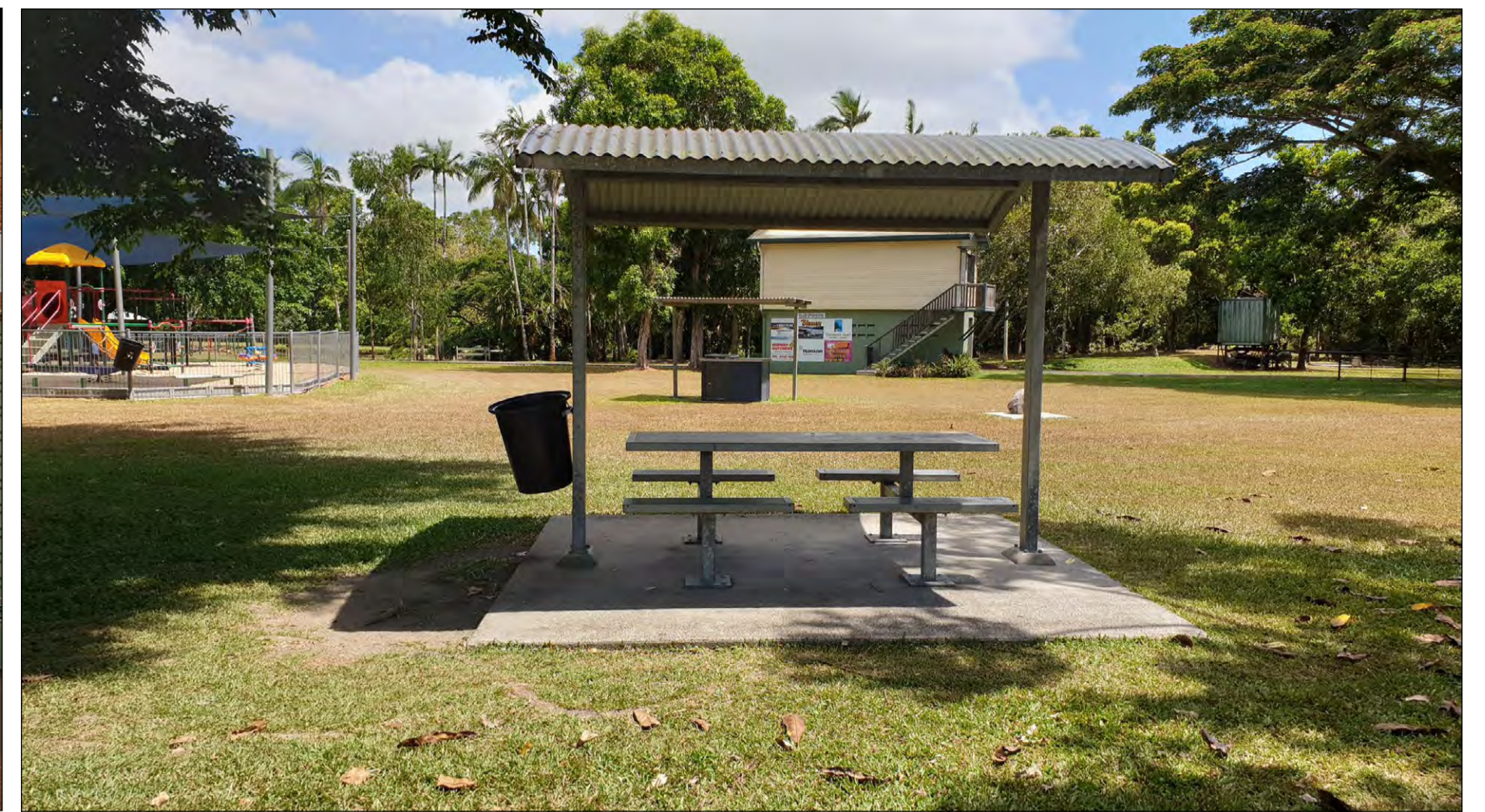
Existing picnic shelters are very unremarkable.
