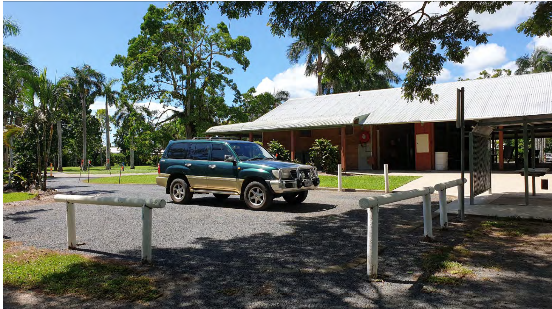
Side carpark near Covered Shed building and BBQ shelter.
