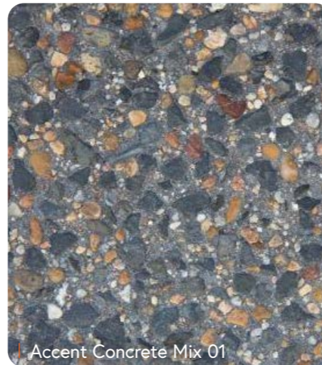
Innisfail CBD Existing Concrete Pavement
